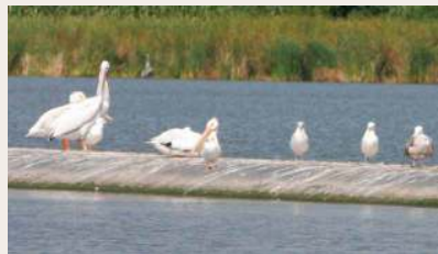
Geotube® Dyke for wetland engineering.
