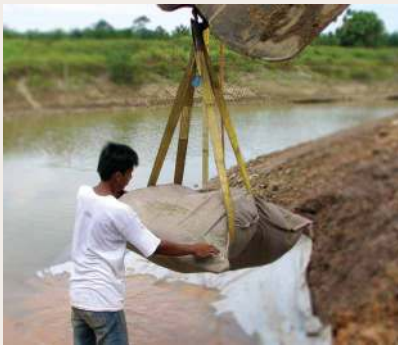
Lifting and positioning Geobag unit.
