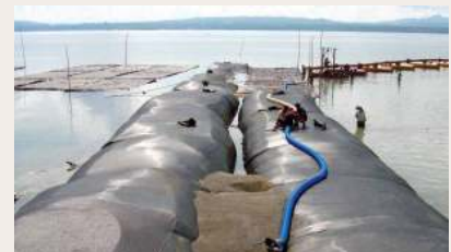
Geotube® Dyke for lakeshore reclamation.
