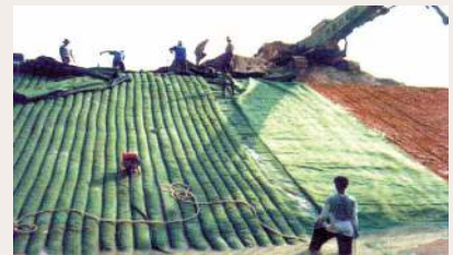
Geotube® Sand Filled Mattress hydraulically with sand.
