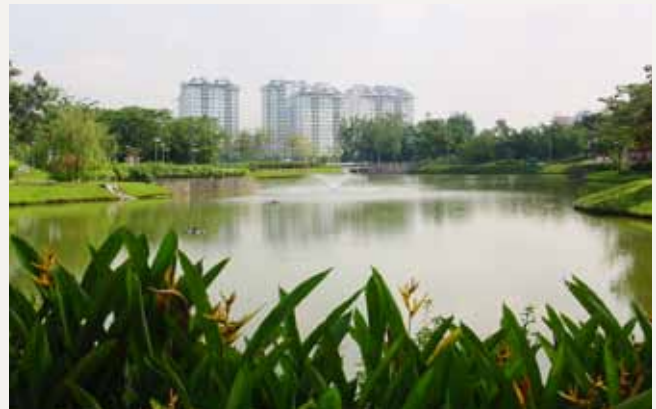
Recreational pond lined with Enviromat® GCL
