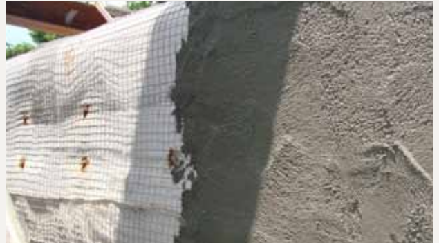
Enviromat® GCL attached to basement wall prior to backfilling
