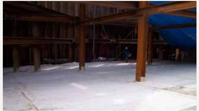
Enviromat® GCL laid prior to casting of basement slab
