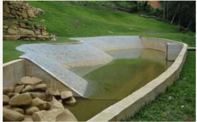
Detention pond lined with Enviromat® GCL
