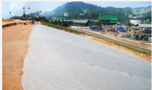
Enviromat® GCL laid over slope
