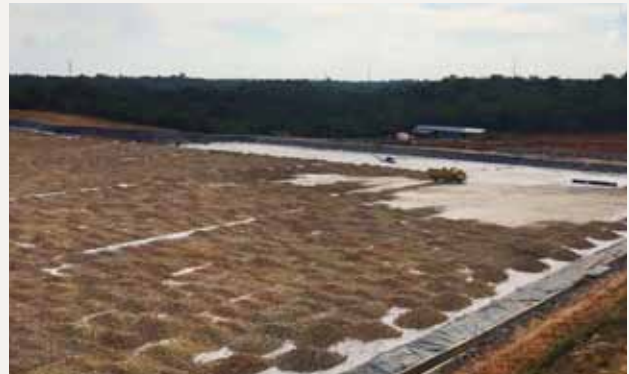
Enviromat® GCL laid as base liner
