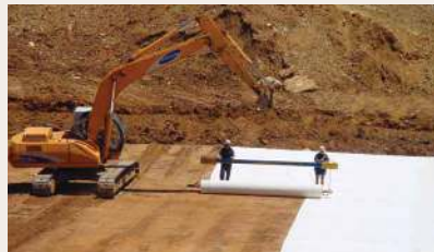
Laying Polyfelt® Enviromat GCL using crane.
