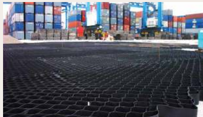
Polyfelt® Envirocell increases the load bearing capacity of subgrades.
