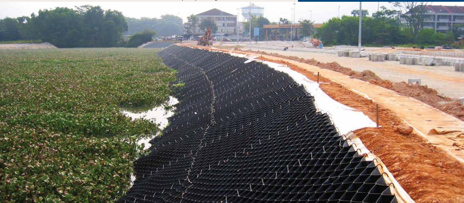
Polyfelt® Envirocell increases the load bearing capacity of subgrades.
