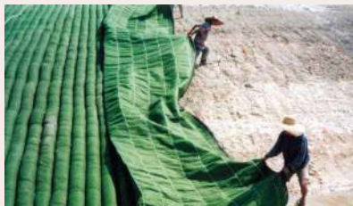
Laying Geotube® Sand Filled Mattress over prepared slope.
