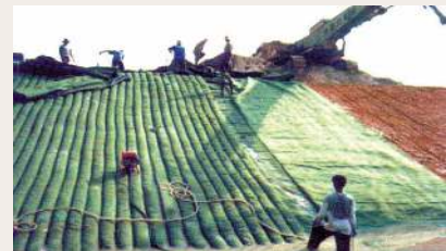
Geotube® Sand Filled Mattress hydraulically with sand.
