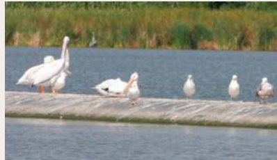
Geotube® Dyke for wetland engineering.
