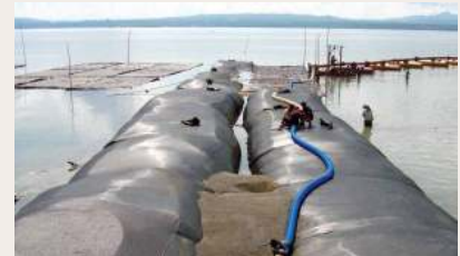
Geotube® Dyke for lakeshore reclamation.
