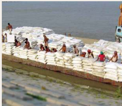
Deploying Geobag units by dropping into water.
