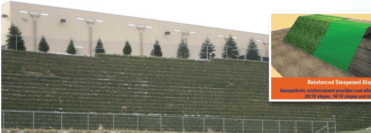
Lowe's Store, Western Hills, OH, Height = 65 1H:3V Miramesh GR inside wire basket wall.
