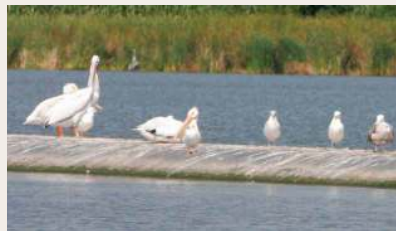
Geotube® Dyke for wetland engineering.
