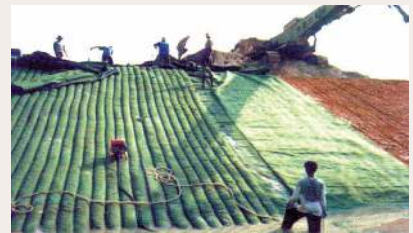
Geotube® Sand Filled Mattress hydraulically with sand.
